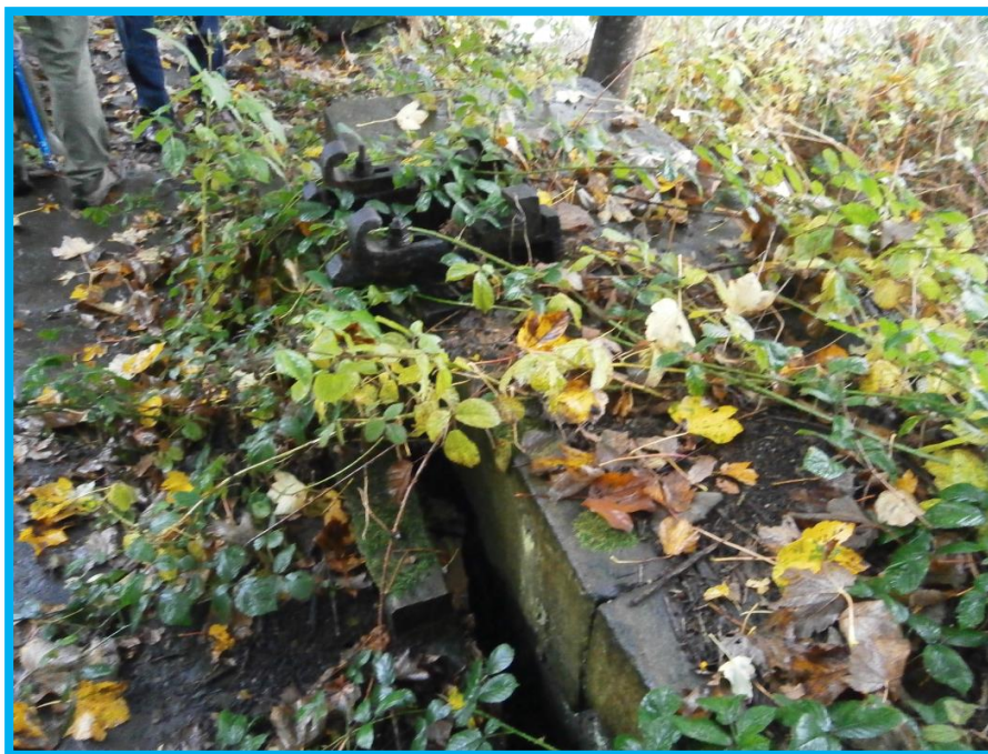
Fig 10 Stone structure with slot for sluices, showing brackets.
