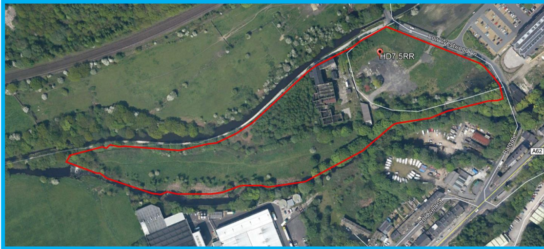
Fig 5 Satellite view of site within red outline. Note extent of buildings. The boundary line is taken from the OS map base, but in reality, the boundary is the centreline of the River Colne, along the length of the site (GoogleEarth).
