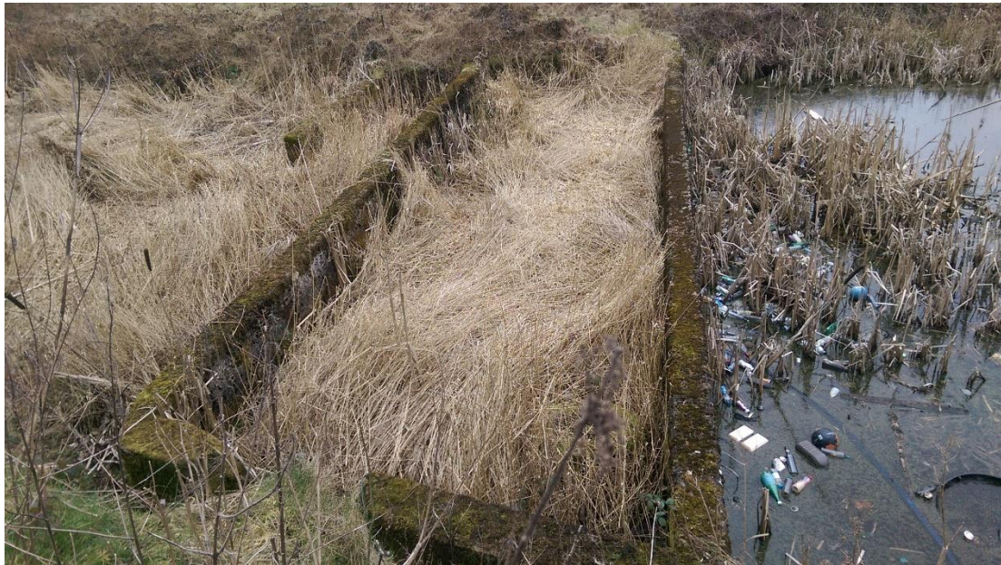
Figure 16 | Mill Race showing wall structures and assumed stilling / clarification pond
