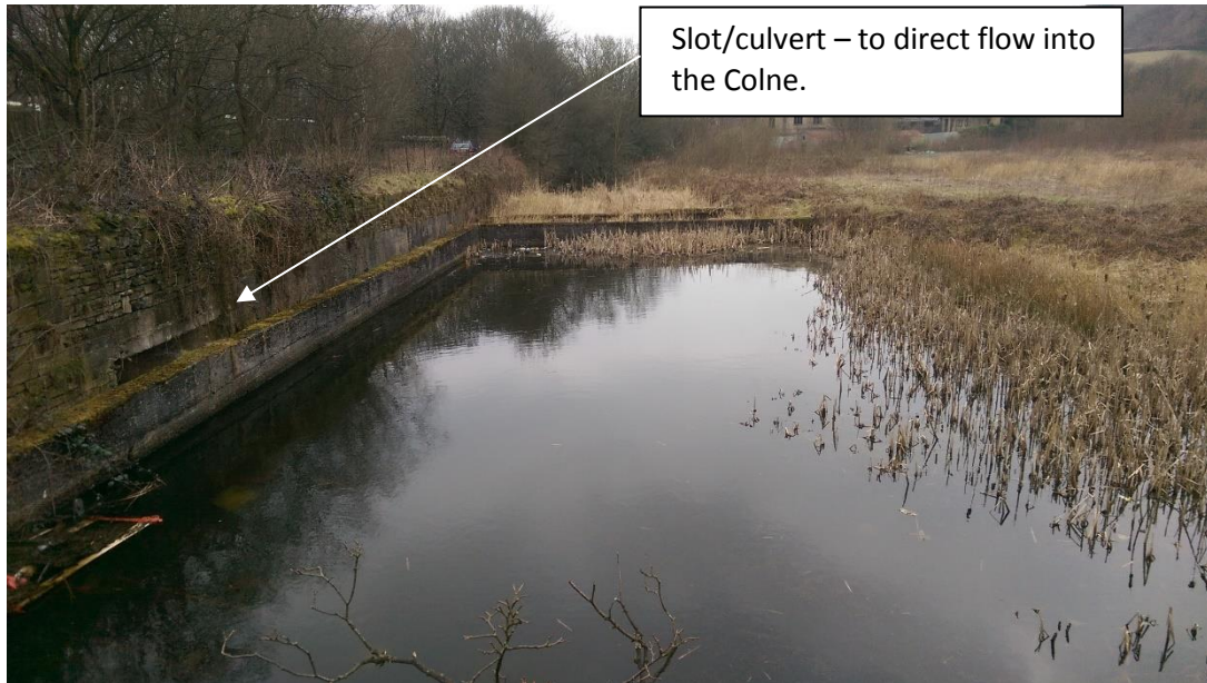
Figure 15 | Mill Race showing wall structures and assumed stilling / clarification pond
