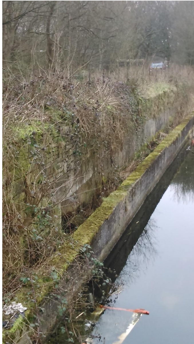
Figure 17 – Channel/ditch running along the mill race. It appears that the walls preferentially direct flow along this route, although this is unconfirmed.
