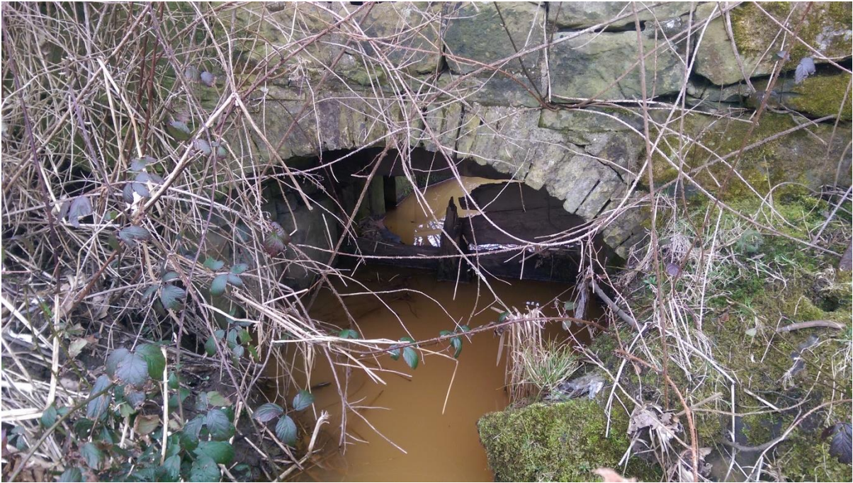
Figure 13 – Arch partially obstructed by deteriorated timber sluice
