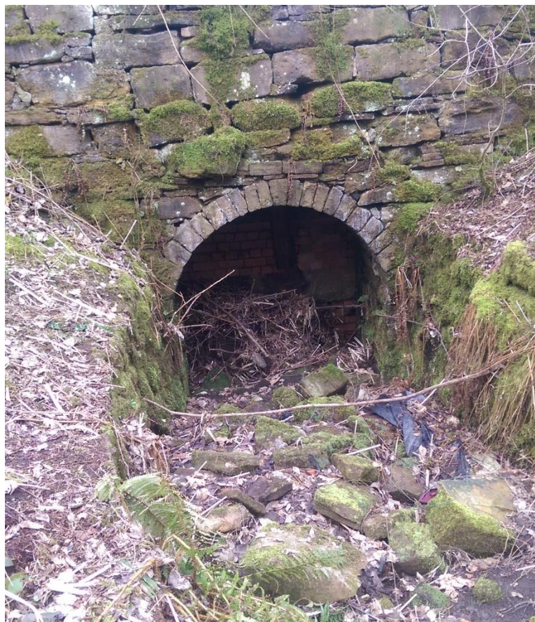
Figure 13 – Arch partially obstructed by deteriorated timber sluice
