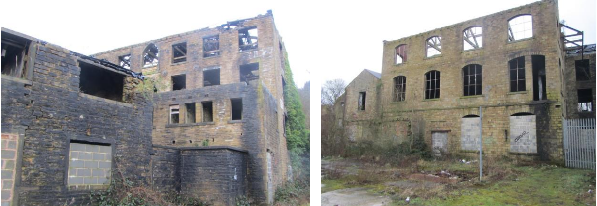
Figure 6 General views of the mill building
