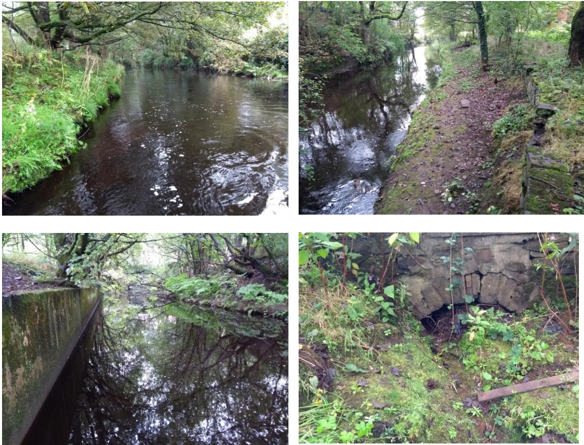
Figure 2(a-d) Typical views of the channel including culvert
